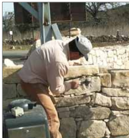
Assistant Vineyard Manager David Maduena and his crew reconstructed the gate
